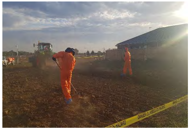
Photo 4. Test pit remediation of Lot 1513, TP46, Lot 1514, TP44 and Lot 1526, TP17
