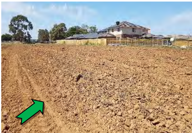
Photo 5. Riverwalk Stage 15 following remediation works.
