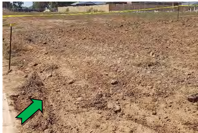
Photo 6. Riverwalk Stage 15 following remediation works
