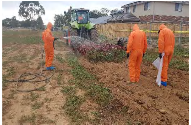
Photo 2. Riverwalk Stage 15 during remediation works.
