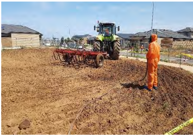
Photo 3. Riverwalk Stage 15 during remediation works
