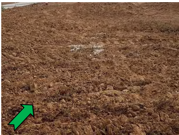
Photo 5. Riverwalk Stage 18 following remediation works.
