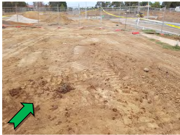
Photo 4. Lot 1809 and 1810, Excavation zone post visual inspection.
