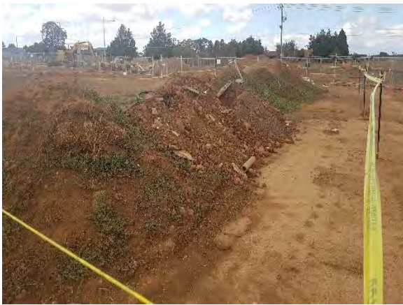
Photo 3. The soil stockpile on Lots 1809 and 1810 prior to removal works.
