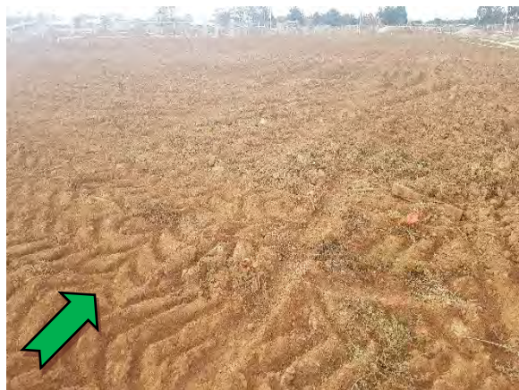
Photo 6. Riverwalk Stage 18 following remediation works.
