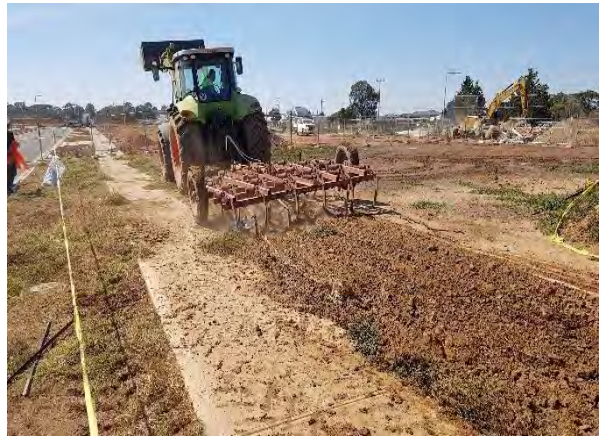
Photo 2. Asbestos-containing fibre cement sheet debris removed from the soil surface within Riverwalk Stage 18.
