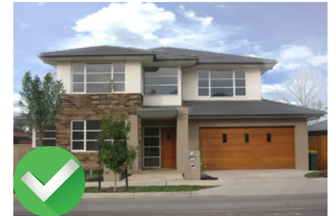
Example of compliant sectional panel lift door, and garage set back behind front facade.
