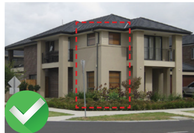
Window with matching head and sill at corner.
