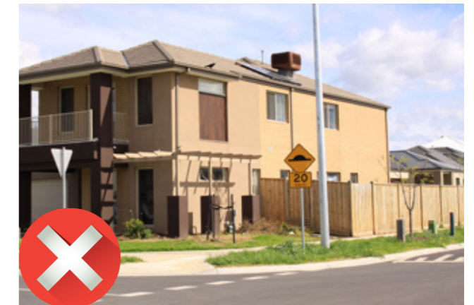
This cooling unit is visible from the primary and secondary streets, and so does not comply.
