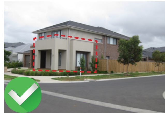
Continuation of front facade to Secondary Street.
