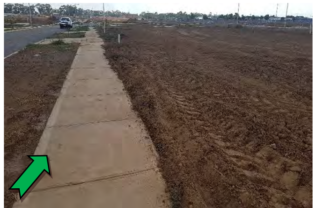
Photo 6. Riverwalk Stage 17 following remediation works.
