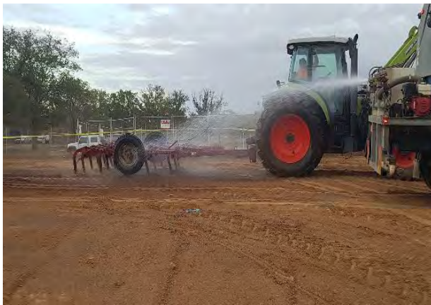
Photo 3. Riverwalk Stage 17 during remediation works.
