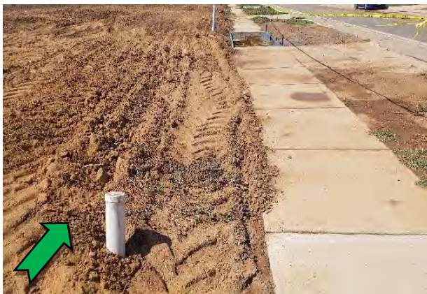
Photo 5. Riverwalk Stage 17 following remediation works.
