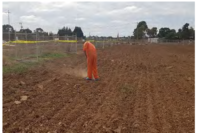
Photo 4. Test pit remediation of Lot 1706, TP46.
