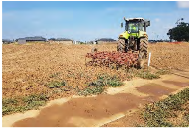
Photo 2. Riverwalk Stage 17 during remediation works.
