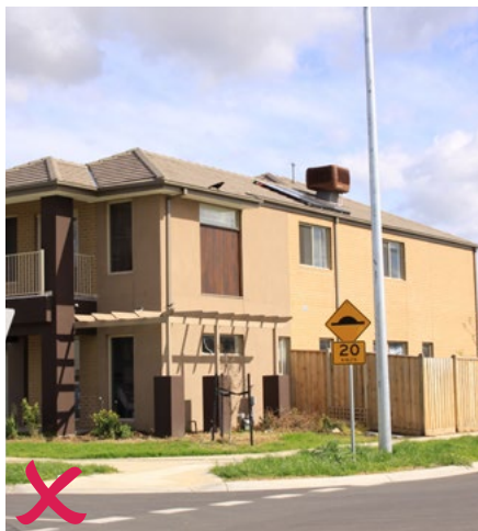
This cooling unit is visible from the primary and secondary streets, and so does not comply.
