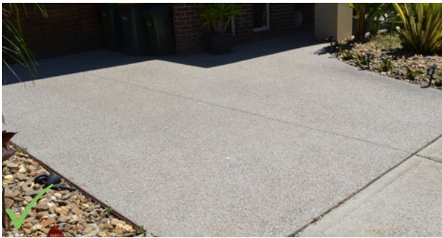
Example of driveway constructed using exposed aggregate concrete.
