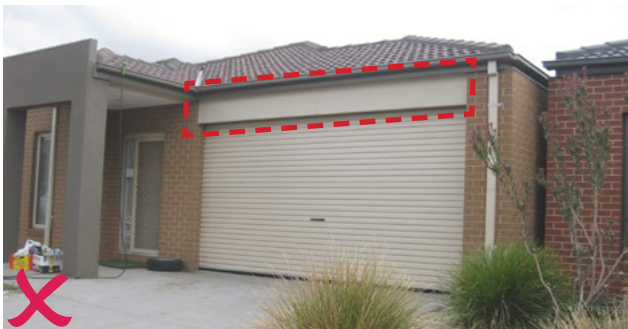
Infill above opening not permitted.
