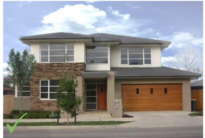
Example of compliant sectional panel lift door, and garage set back behind front facade.
