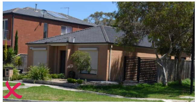
Roll down security shutters are not permitted where visible from public area such as street frontage, or reserves or parkland.
