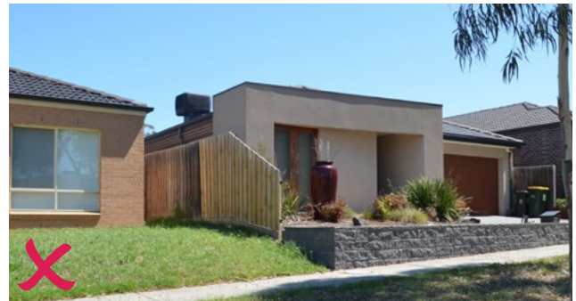
Interlot fencing must not be forward of the building.
