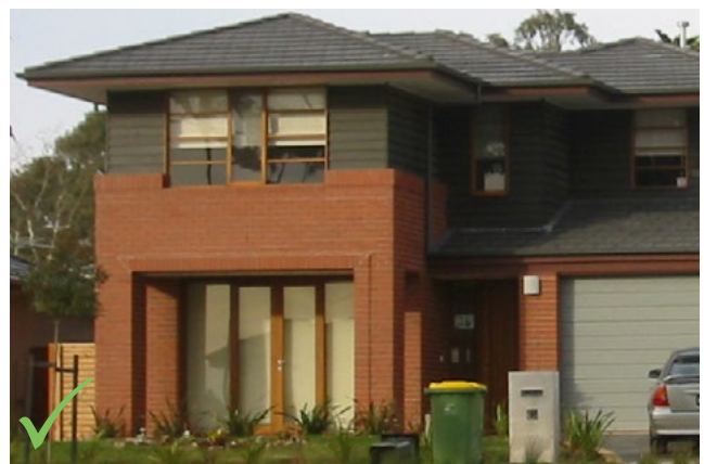
North facing habitable room windows and glass doors should have a minimum 450mm eave or fixed top projection.
