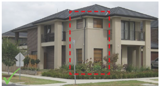
Window with matching head and sill at corner.
