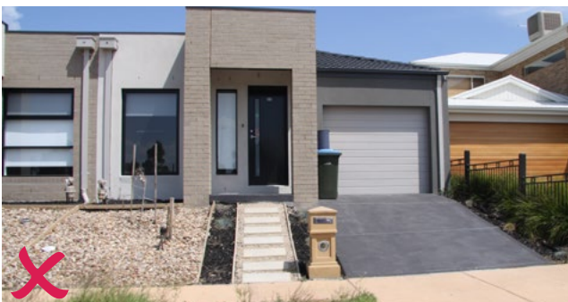
Example of driveway colour and finish not permitted.
