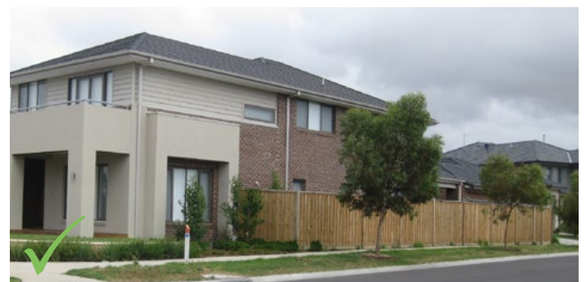
Timber paling fencing on Secondary Street setback at least 3.0m behind the front building line.
