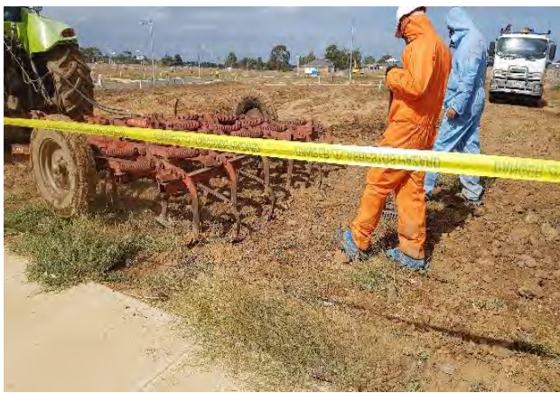
Photo 3. Riverwalk Stage 16 during remediation works.
