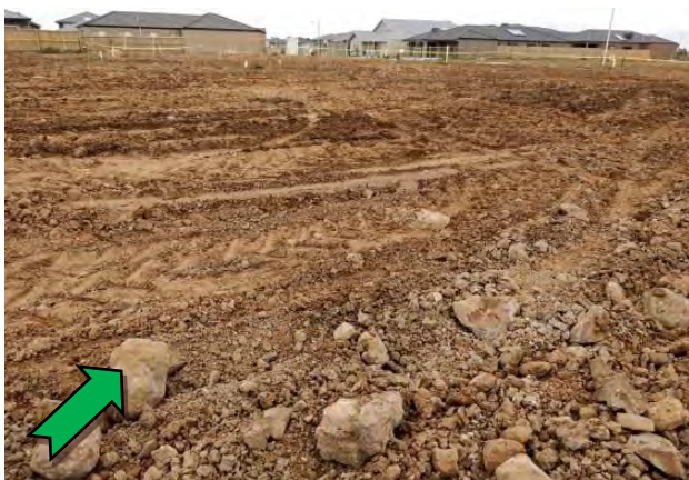
Photo 5. Riverwalk Stage 16 following remediation works.
