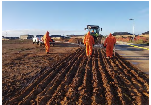
Photo 2. Riverwalk Stage 16 during remediation works.
