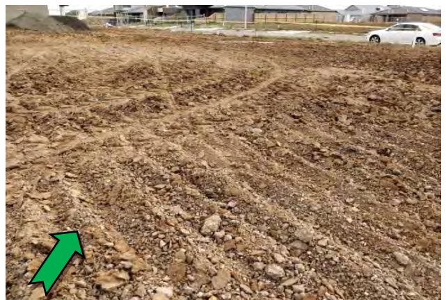
Photo 6. Riverwalk Stage 16 following remediation works.
