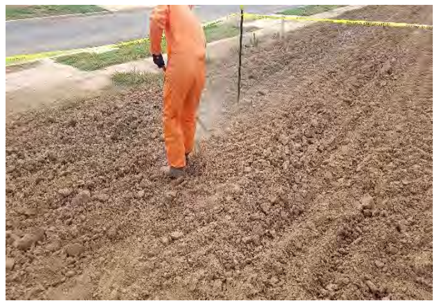
Photo 4. Test pit remediation of Lot 1630, TP16.
