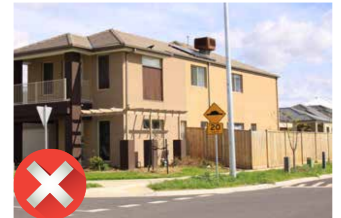
This cooling unit is visible from the primary and secondary streets, and so does not comply.
