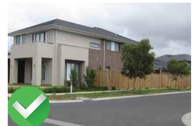
Timber paling fencing on Secondary Street setback at least 3.0m behind the front building line.
