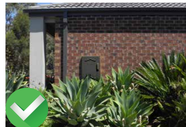
Example of meter box on side of house screened by planting and painted to match the downpipe and house.
