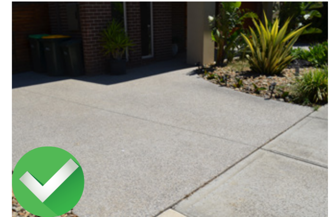
Example of driveway constructed using exposed aggregate concrete.
