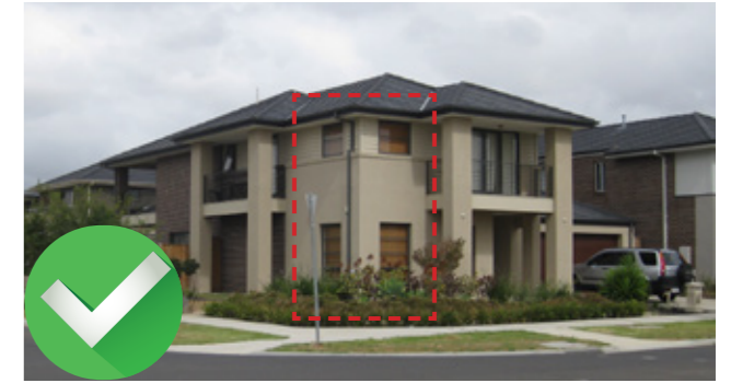
Window with matching head and sill at corner.
