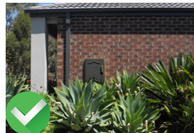
Example of meter box on side of house screened by planting and painted to match the downpipe and house.
