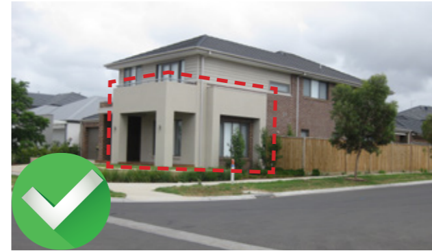
Continuation of front facade to Secondary Street.
